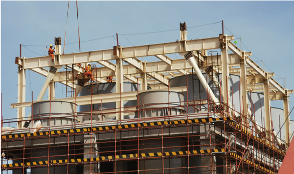
高空作业安全绳拉设规范 Specification for Safety Rope Drawing for Aerial Work
